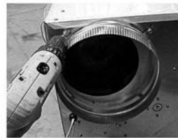
Figure 4: Installing exhaust collar.
