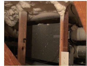
Energy Recovery Ventilator installed in the home.
