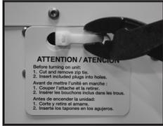
**⚠ CAUTION! REMOVE COMPRESSOR SHIPPING TIE FROM THE UNIT. FAILURE TO REMOVE SHIPPING TIE WILL CAUSE EXCESS VIBRATION TO BE TRANSMITTED TO THE FRAME.**
